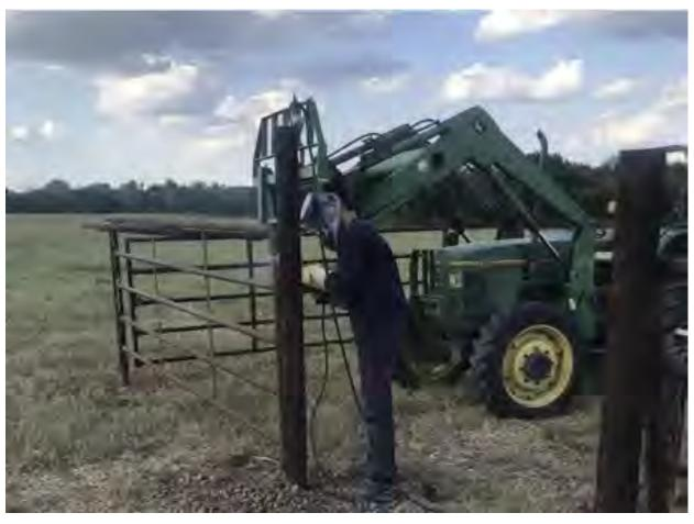
I am welding a section of continuous panels to make our new lot. I am wearing an autodarkening helmet to protect my eyes and a fire-retardant shirt and gloves. I also am wearing leather shoes and a pair of jeans to protect my feet and legs from sparks and spatter.
